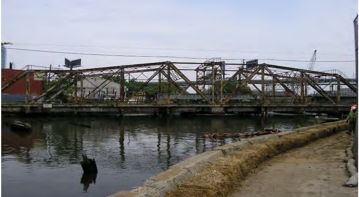
Figure 4: Southern LIRR NYC Rail Freight Bridge - "DB" Bridge
